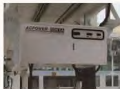
Airport Apron / Hangar
