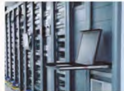
Control Room/ Data Center
