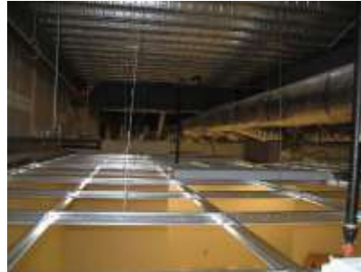
FIG. 7 - Be sure the suspension wires are securely fastened.
