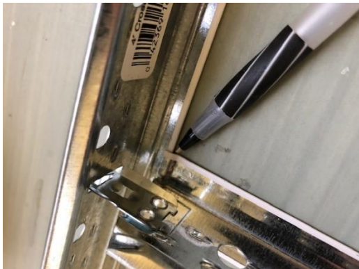
Cross Tee to Main Beam Intersection
