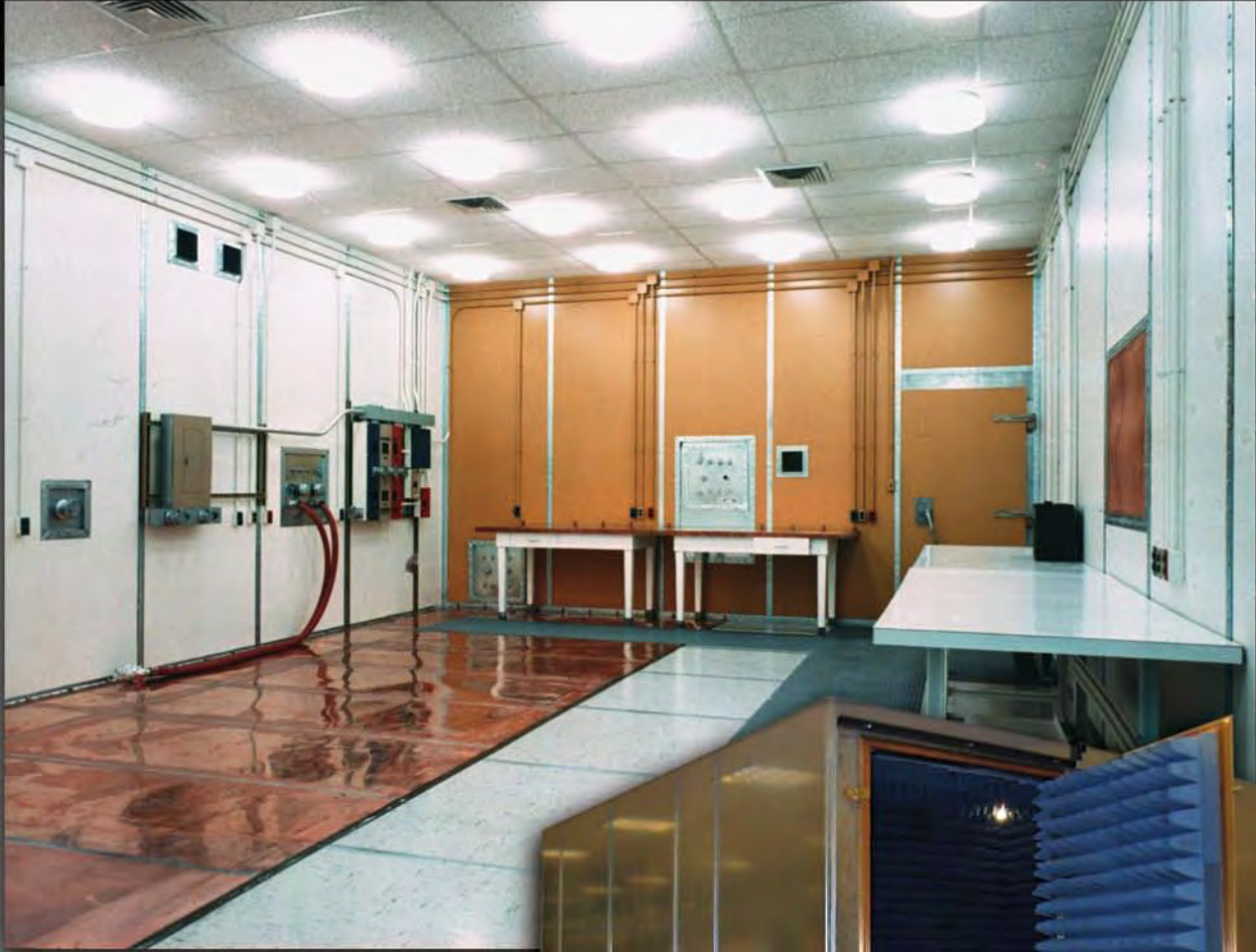
USC Turnkey Installation
