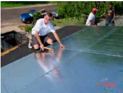
Roof installation gives significant shielding
