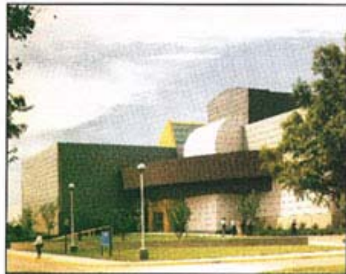
Figure 1. The FAA Registry Building in Oklahoma City, Oklahoma.
