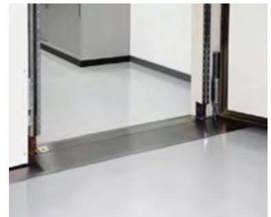
The opening is sealed to provide a barrier-free floor.
