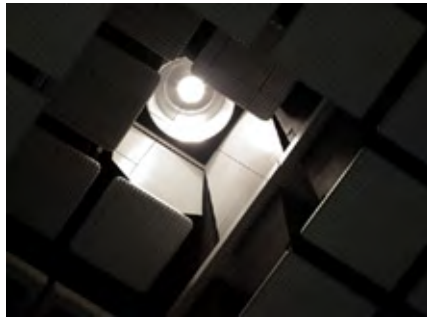
The lighting fixtures are installed deep in a box space which is surrounded by electromagnetic wave absorbers and far enough away for the waves to reach them.
