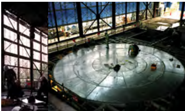
View of large turntable installation ( \phi 3m/10m Dual type, Withstand weight : 30t)
