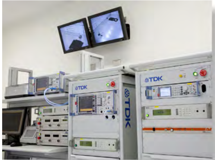
EMC automated measurement system
